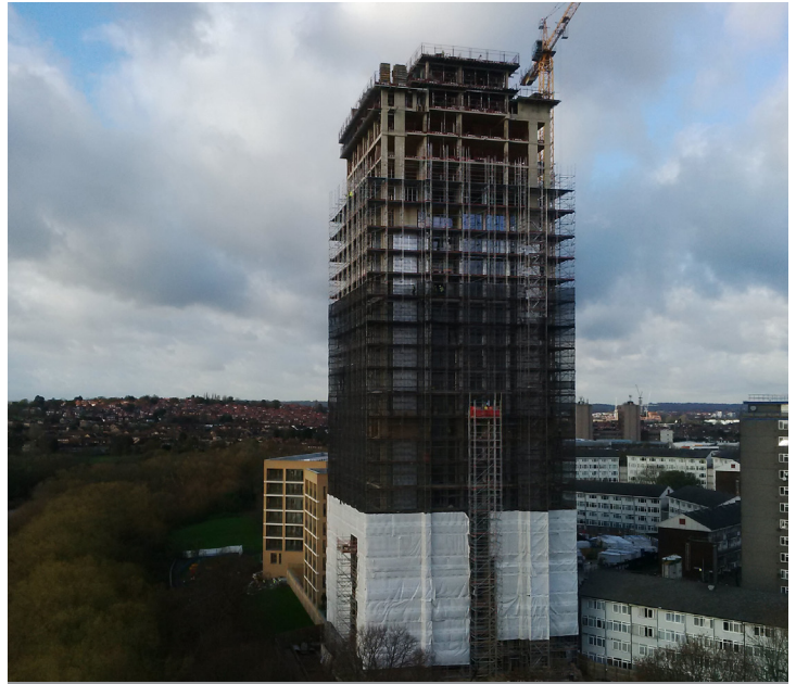
Construction of Block E2
