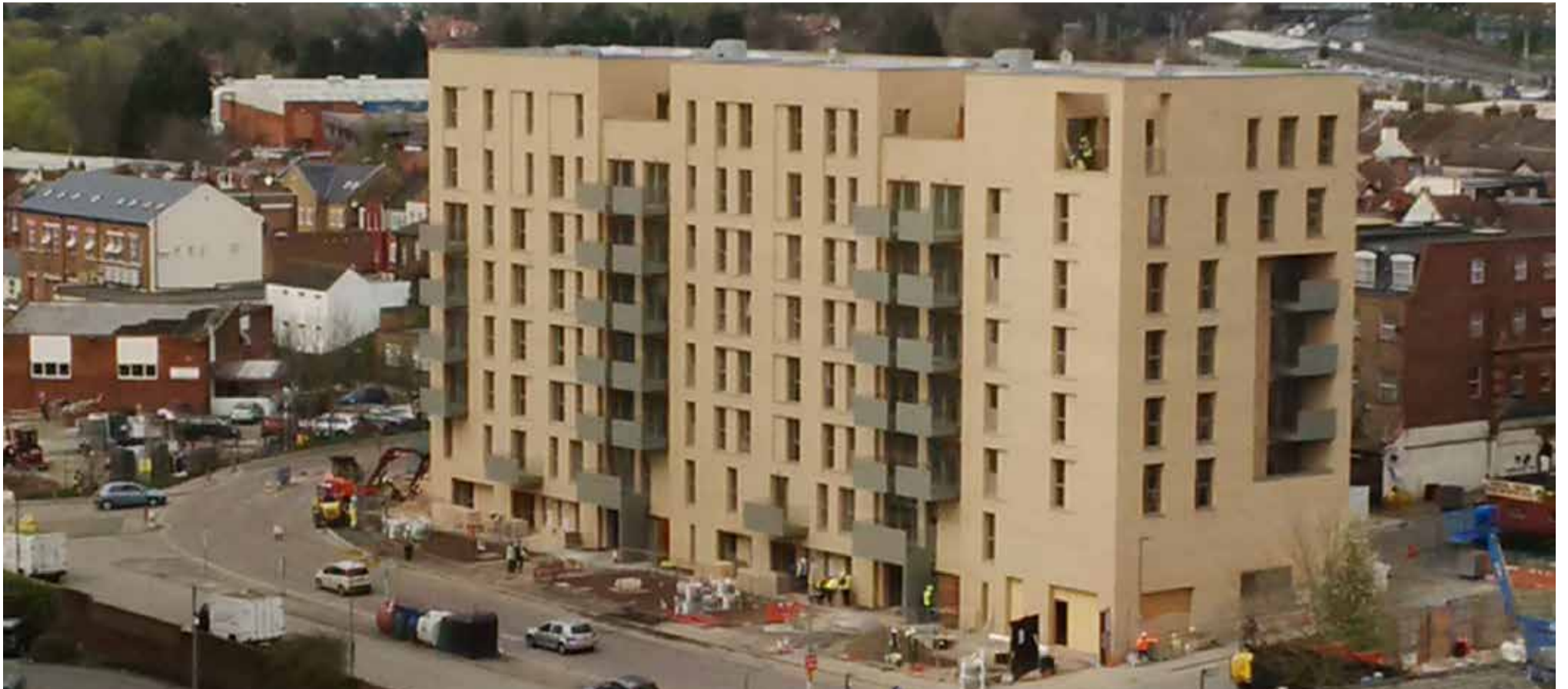
Block G is now complete
