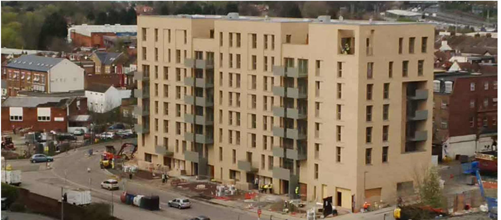
Block G is now complete
