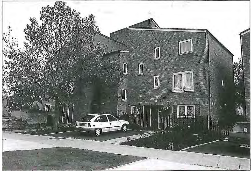
Notting Hill Housing Trust's Adastral development – part of our regeneration programme for Grahame Park
